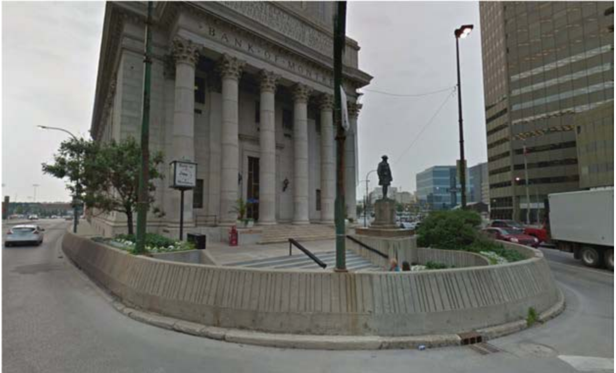
Figure 22 – Depressed Patio Area on SE corner
